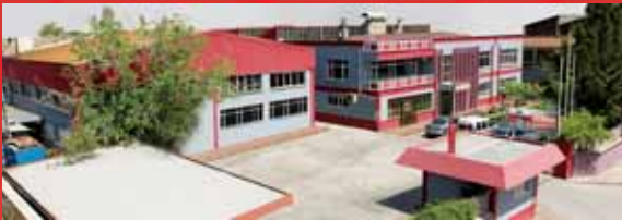
Cylinder Liner Production Facility Motor G mleđi Fabrikası
