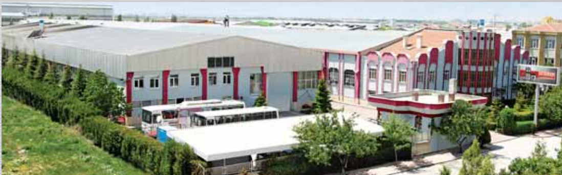
Piston & Piston Pin Production Facility
