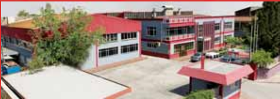
Cylinder Liner Production Facility Motor G mleđi Fabrikası
